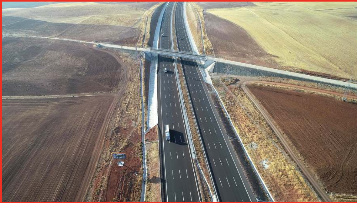
Km: 5+200 Overpass Bridge
