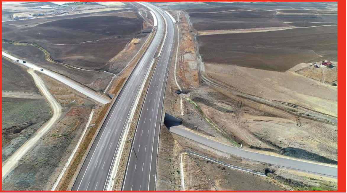
Km: 32+592 Soğulcak Bağıcı Village Underpass
