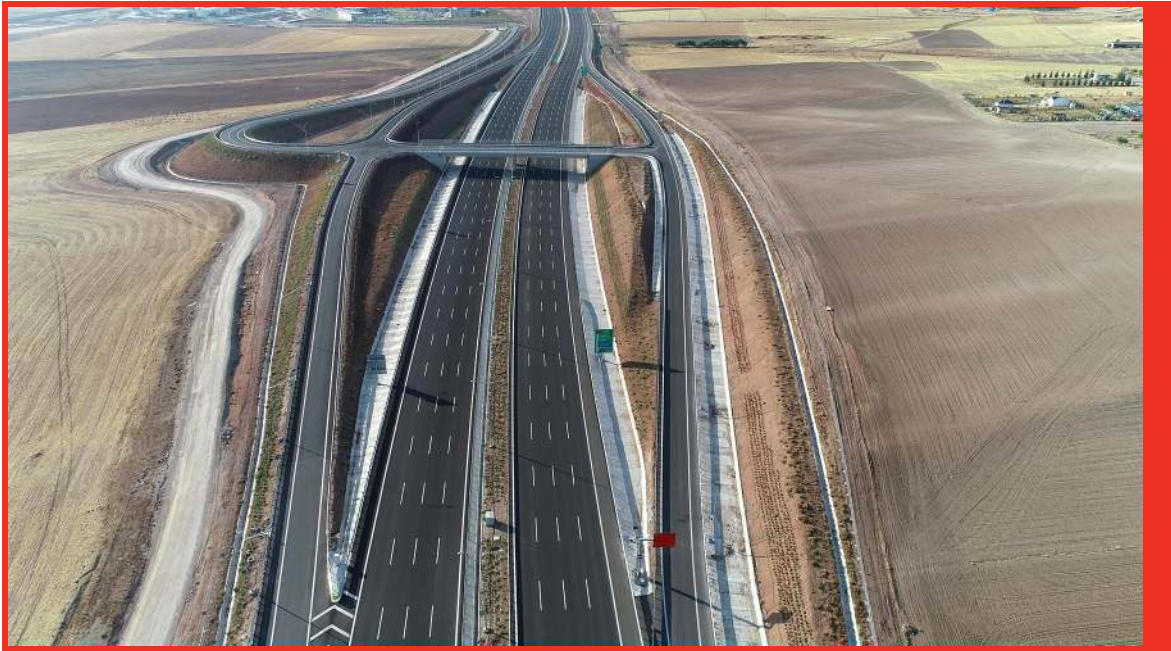
Km: 11+780 Main Command Center Junction
