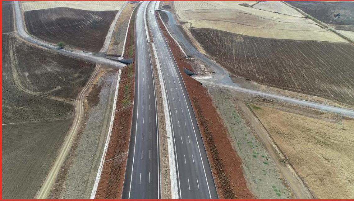
Km: 41+164 Koçyayla-Ahmetçayırı Village Underpass
