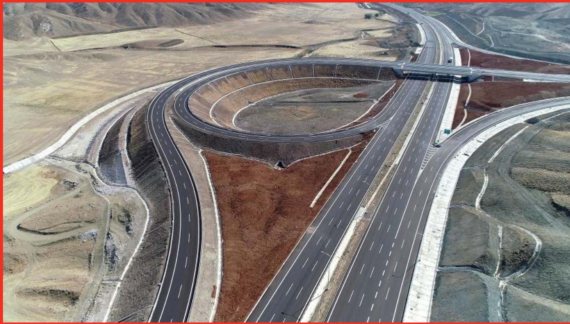
Km: 51+880 Emirler Junction
