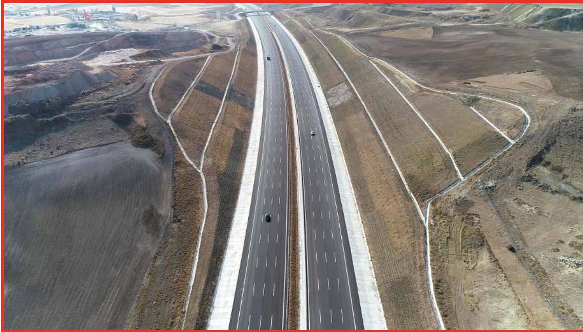
Km: 25+000 Trench Cut
