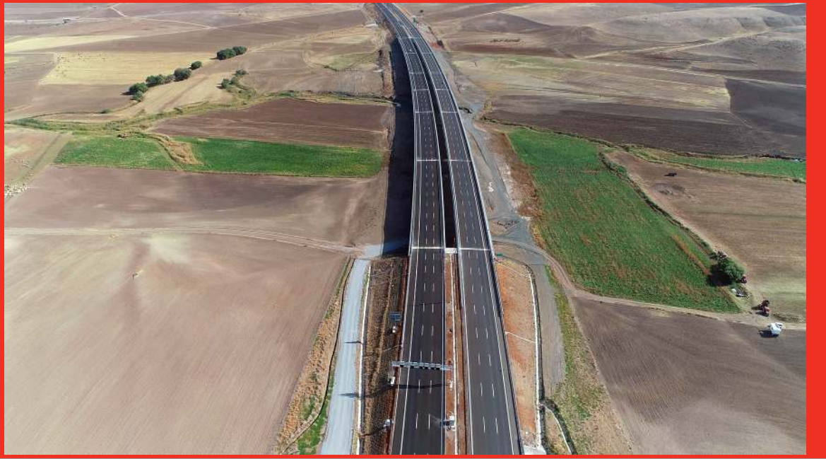
Km: 71+500 Sofular Viaduct
