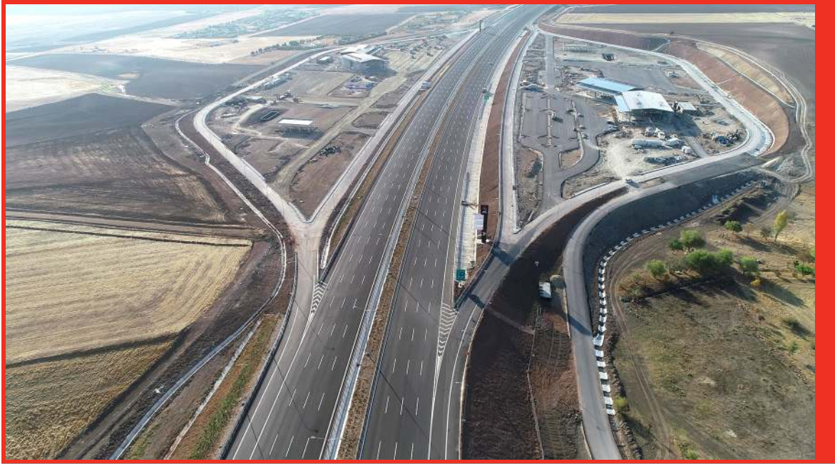
Km: 10+564 Highway Service Facility
