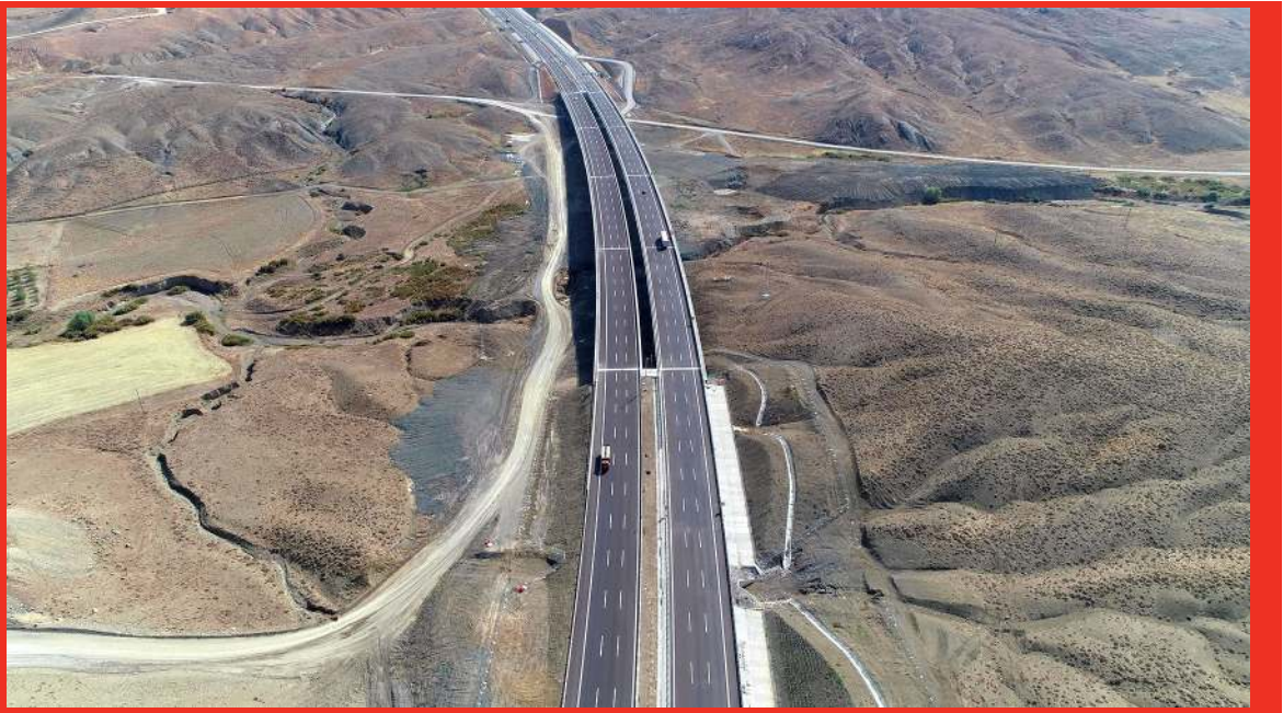
Km: 59+000 Derekışla Viaduct
