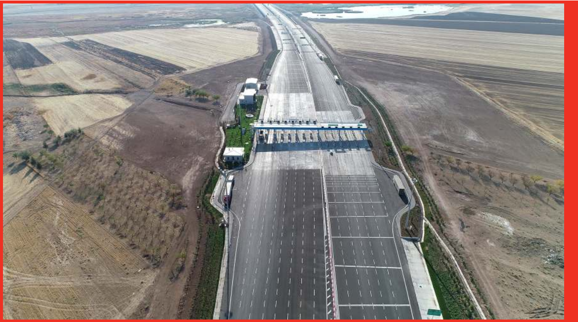
Km: 16+124 Main Toll Plaza
