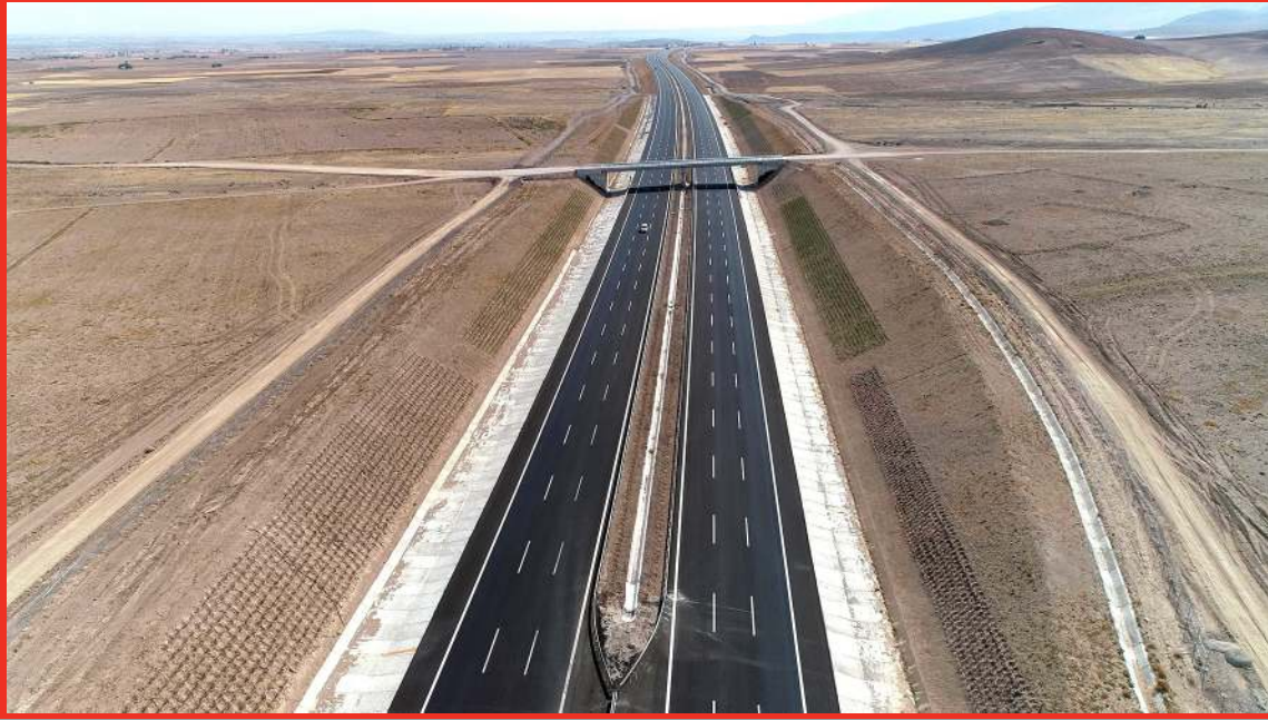
Km: 251+000 Overpass Bridge
