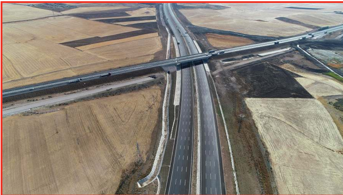
Km: 27+500 Overpass Bridge
