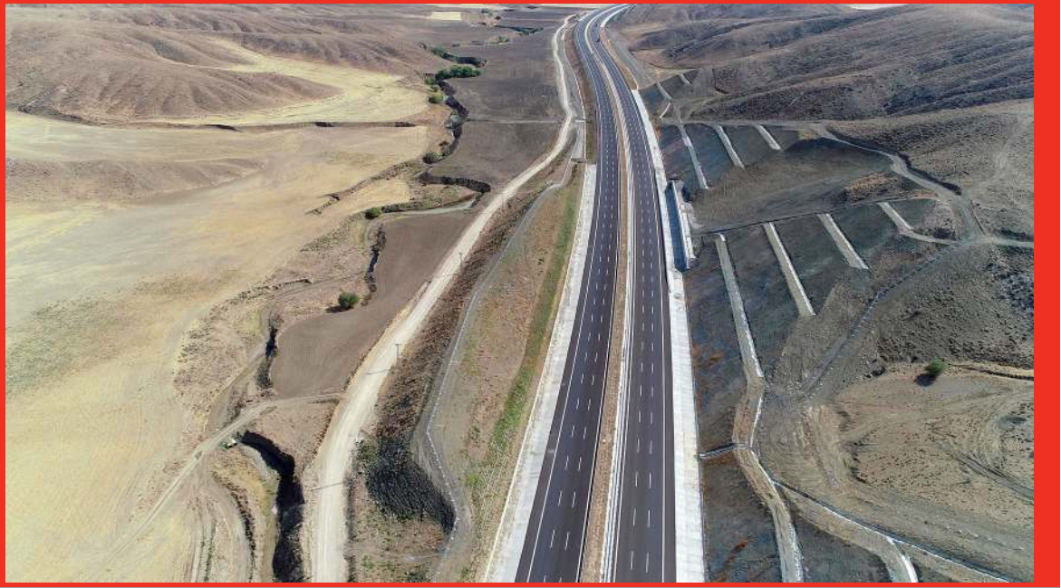
Km: 52+500 Retaining Wall At Cut Section
